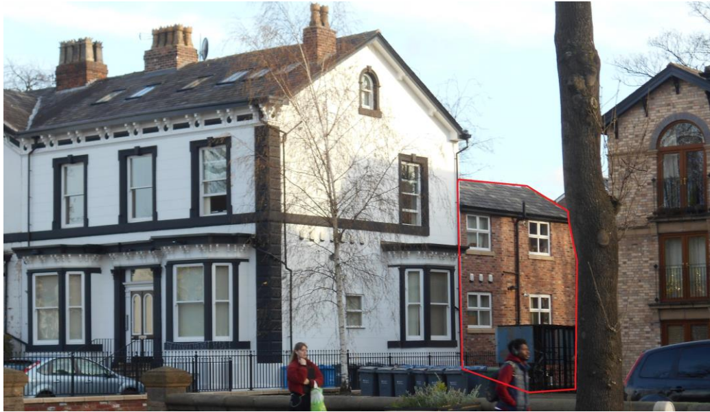
The unauthorised extension when viewed from Wilmslow Road
