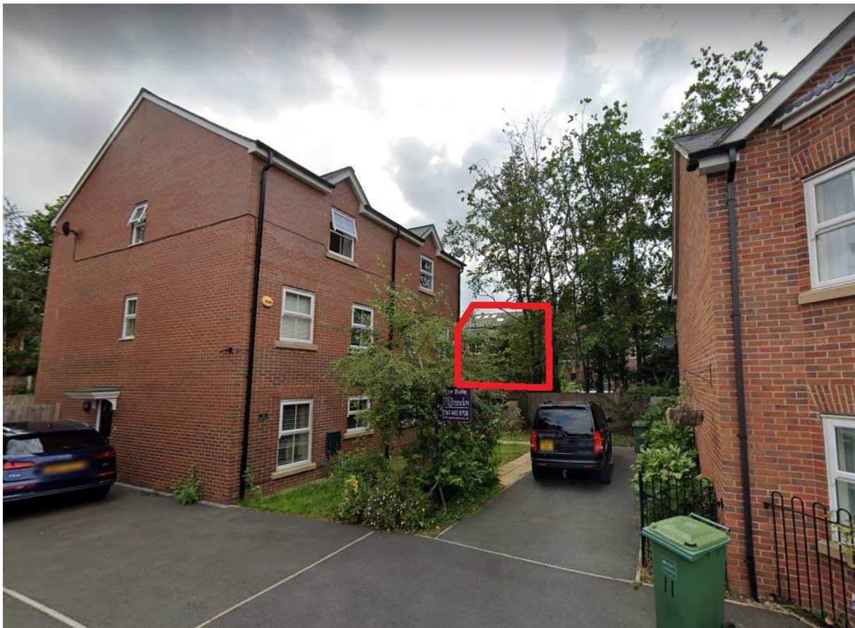
View south west from the head of Besford Close cul-de-sac towards rear of application property edged red
