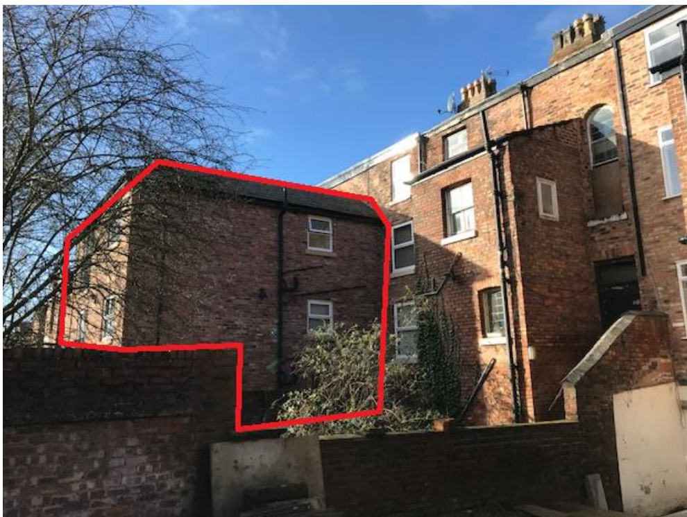
Unauthorised rear extension as viewed from neighbouring property
